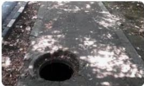
Sewage network without cover in circulation road [3]
